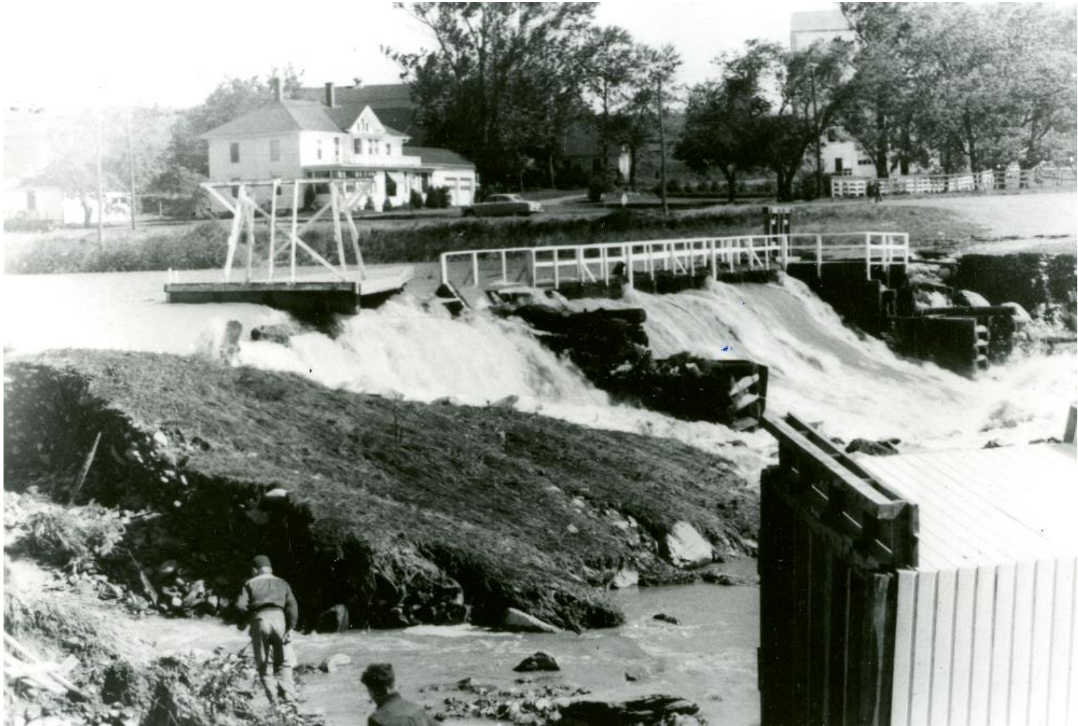
Damage to dam in Limestone, ME
