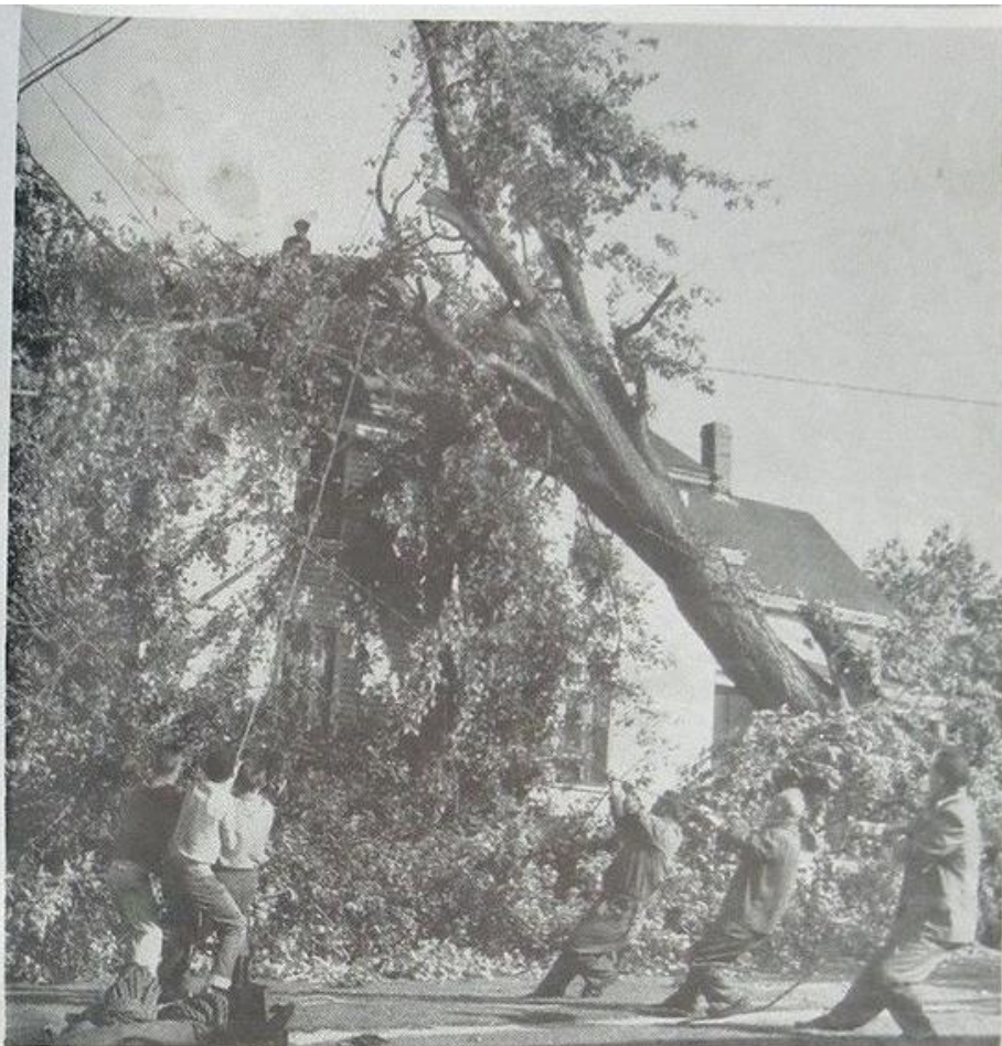
Workmen speedily haul a giant elm from the rooftop of a Portland home after Hurricane Carol had wreaked havoc in Maine's biggest city. Scenes like this were typical throughout the state on Sept. 1, day after the big storm.
