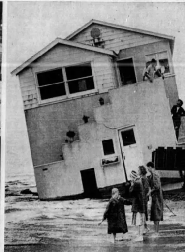
TOPFLING INTO SEA —One of the many beach homes which were destroyed by the heavy surf which undermined foundations in this home on shore of Alamitos Bay. Residents of the home are shown as they removed furnishings as pounding swells shook the dwelling, threatening to topple the damaged structure into the surf. Photo West Jones
