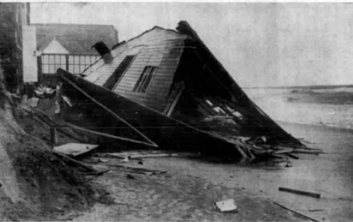
BATTERED BY WAVES —Once a shoreline residence on E. Ocean Blvd., Long Beach, this pile of wreckage indicates the force of the ripping waves that battered at Southland coastline, wrecking scores of homes. Times photo
